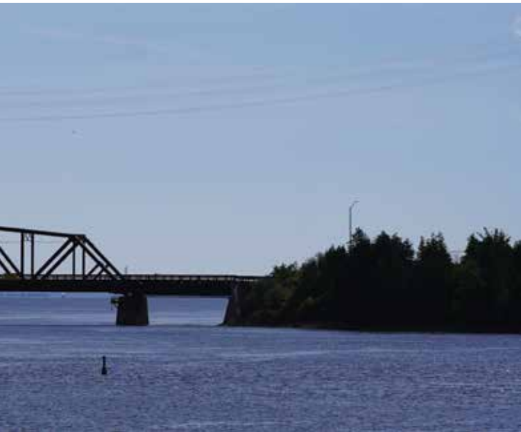
▼ The Swing Bridge, formerly a single-lane rail bridge and the only land connection to the island, in the North Channel at Little Current. When needed, it swings open once an hour to permit tall ships through.
